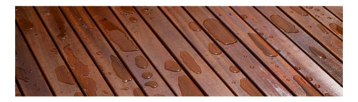
**Stained wood:** The wax and/or silicone in wood preservatives and in water-repellent semi-transparent stains could cause a lack of adhesion. Sanding the surface with No.60 or No.80 sandpaper is therefore strongly recommended.
